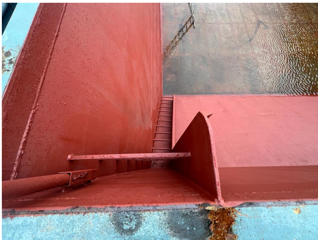
New stairs made to enter cargo area
